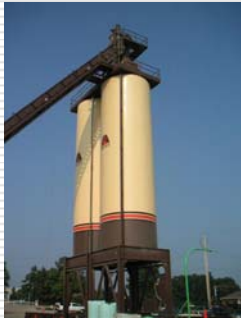
HMA storage silo
