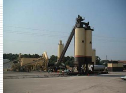
Astec plant located in Alabama
